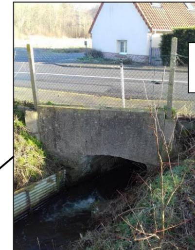
Busage ARMCO sous la RD, 1200mmx1000mm
